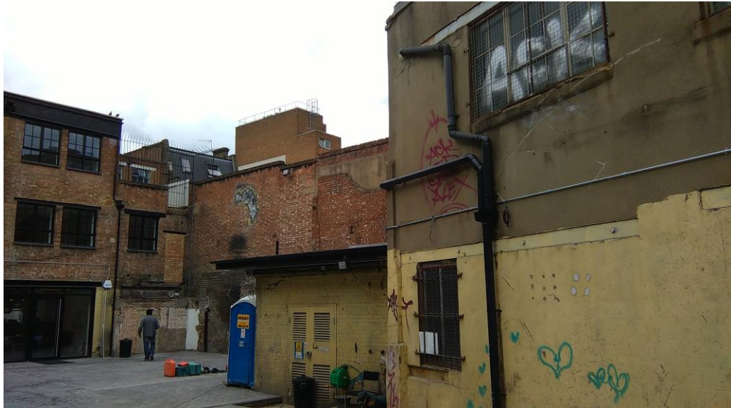
Service Yard looking west
