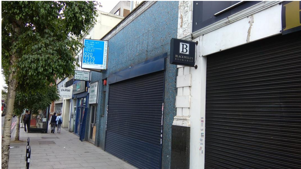
Existing Holloway Road shopfront
