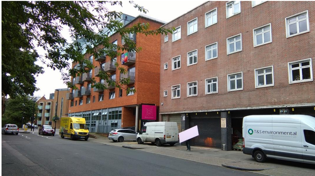
Looking south along Benwell Road
