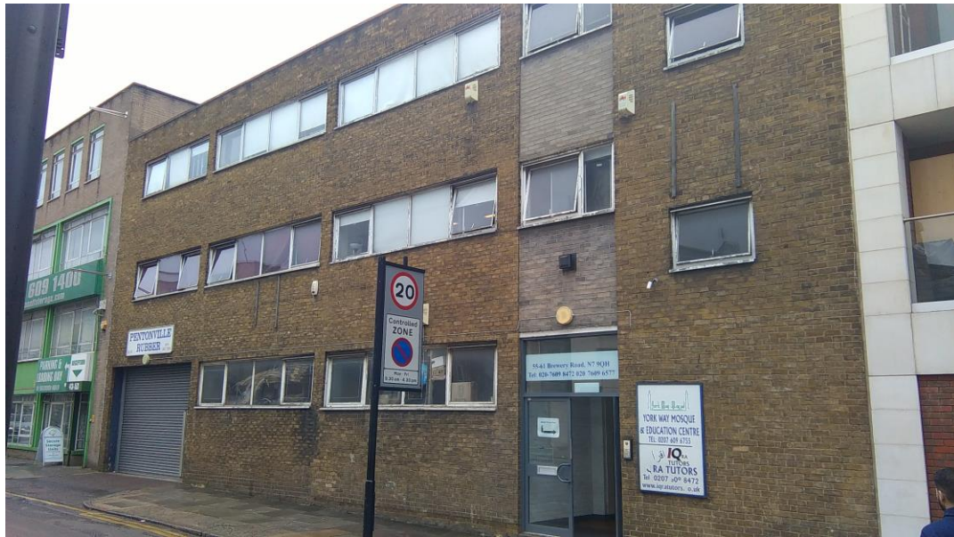
Photograph 2: Existing front elevation
