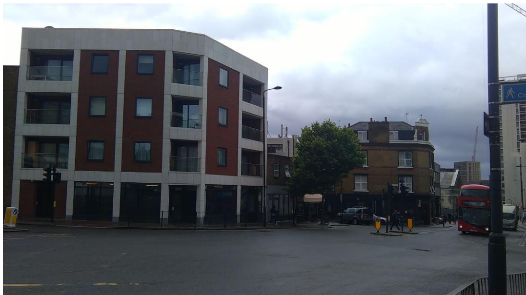
Photograph 3: York Way looking south
